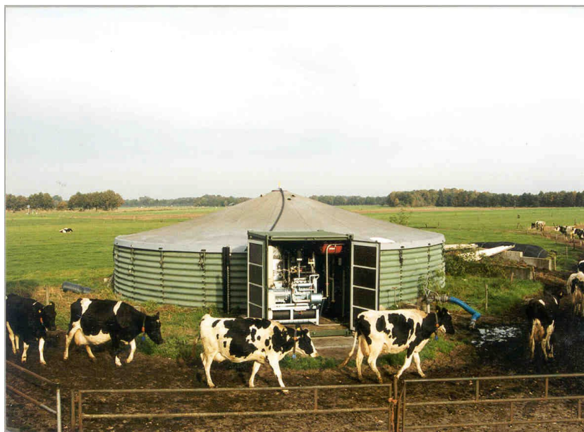
Figure 13 Small scale anaerobic digestion installation. Source BTG
